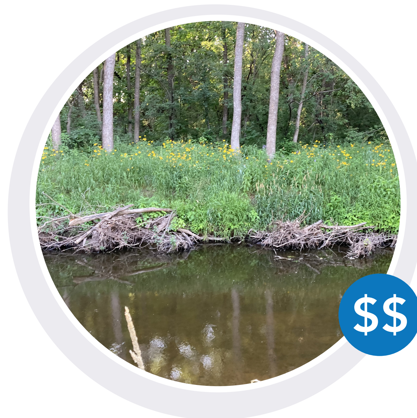
Bank stabilization with bioengineering methods
