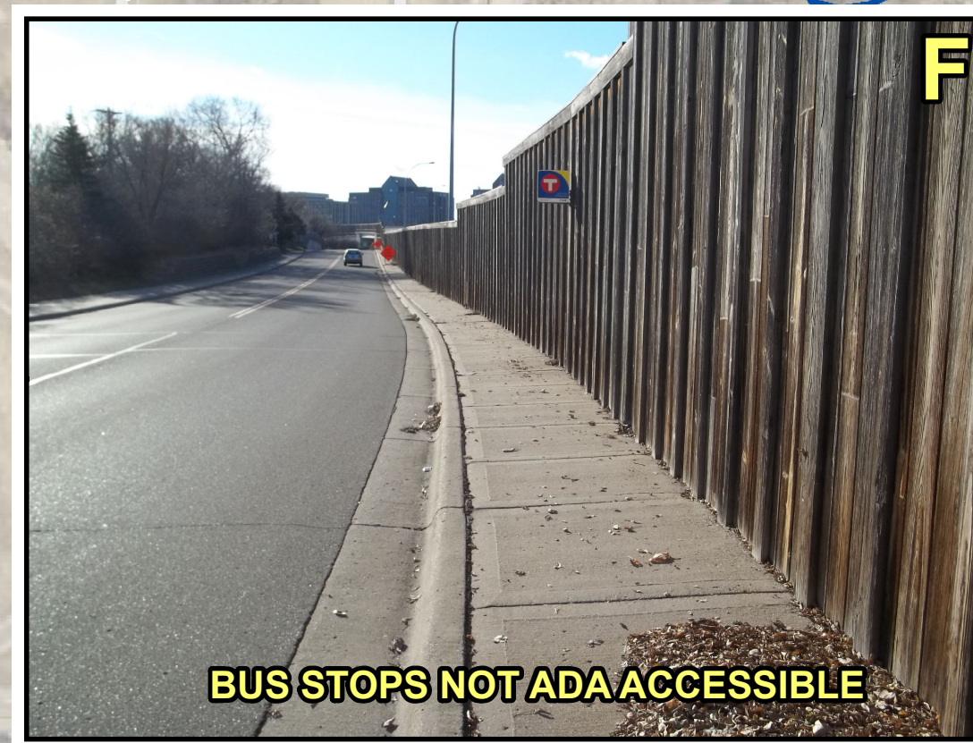
BUS STOPS NOT ADA ACCESSIBLE
