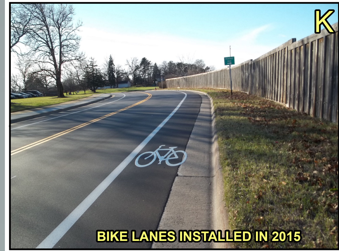
BIKE LANES INSTALLED IN 2015
