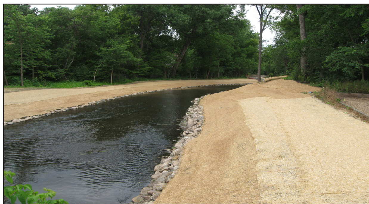
Bassett Creek restoration: bank stabilization and revegetation
