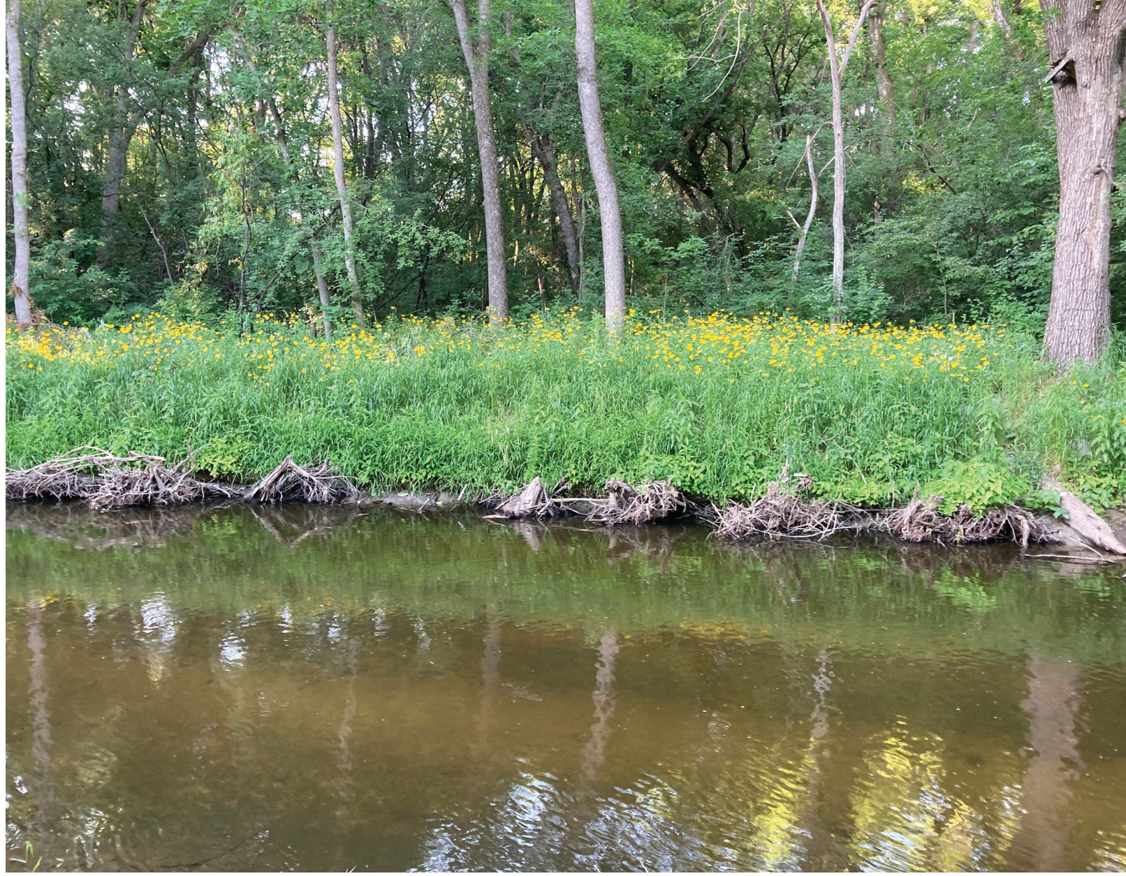
Toe Wood with VRSS and Grading
