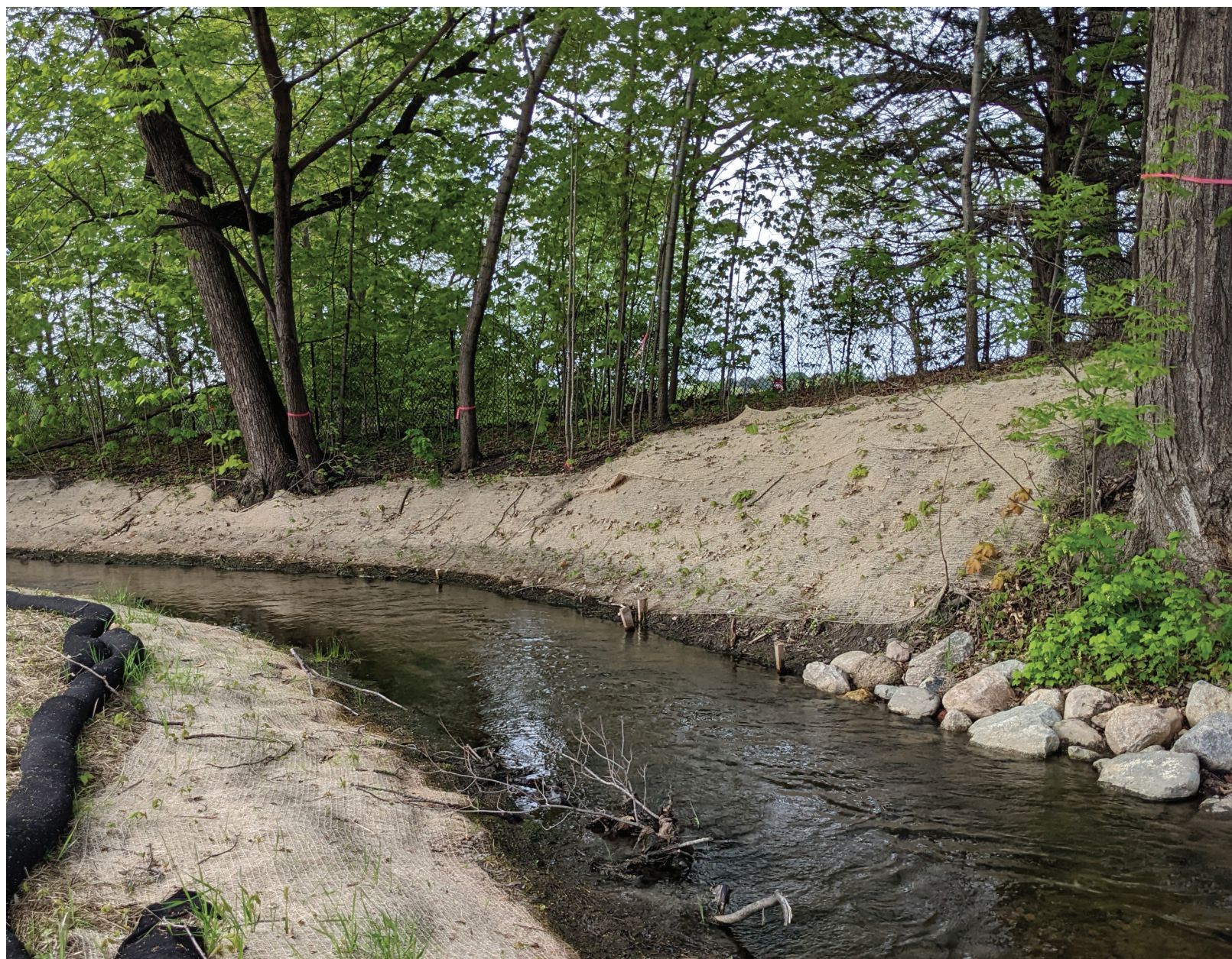
Coir Log with Bank Grading
