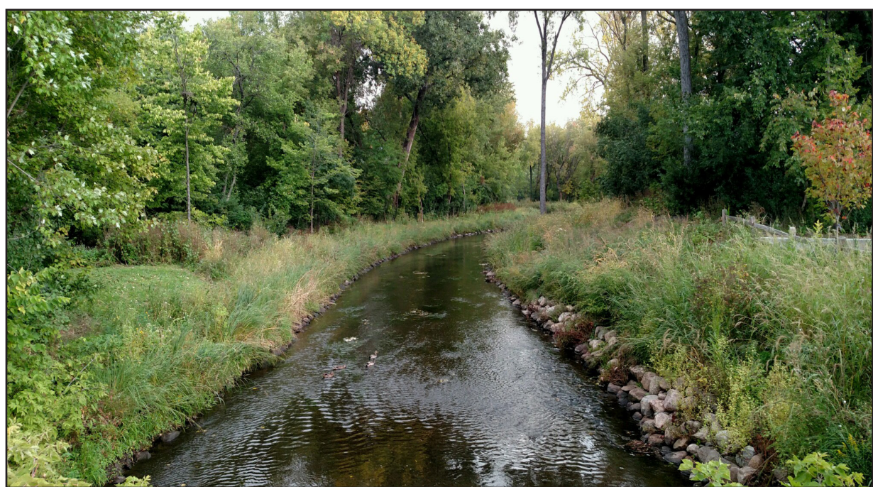
Bassett Creek restoration: bank stabilization and revegetation
