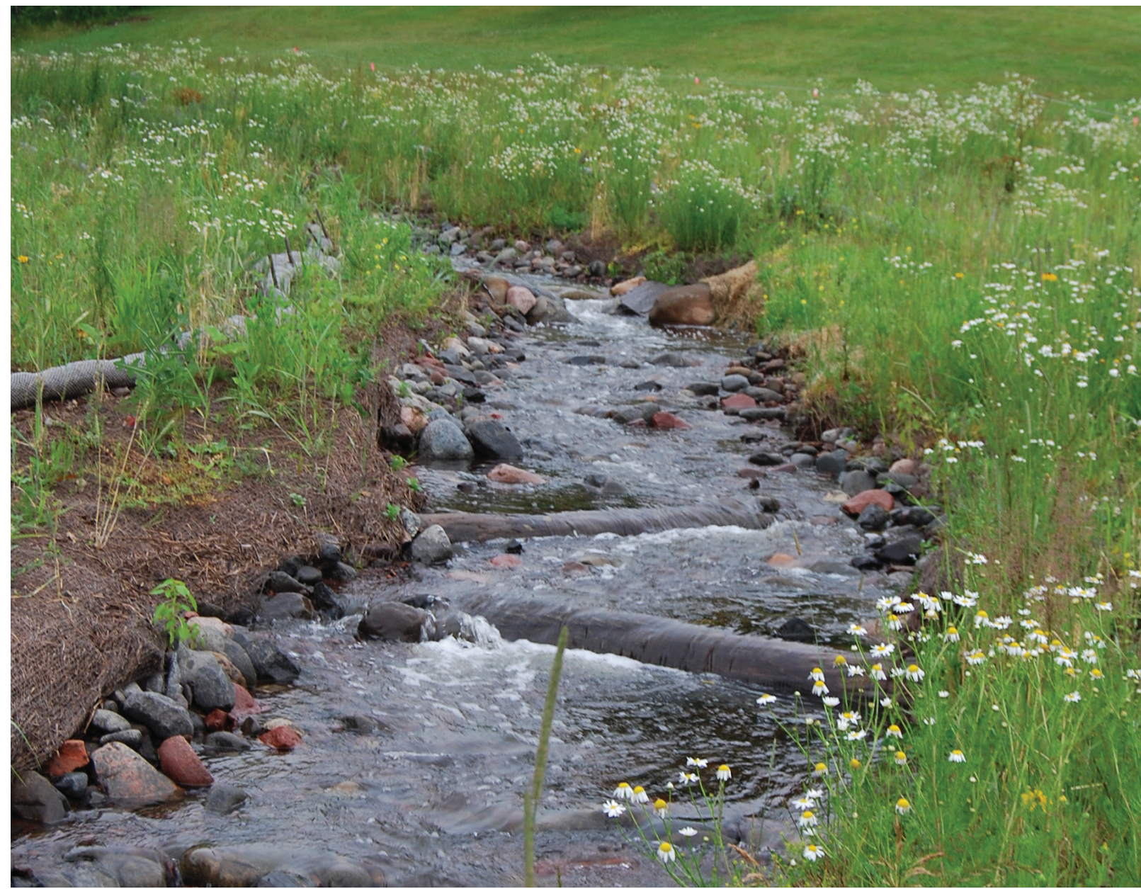
Rock Toe with Log Vanes
