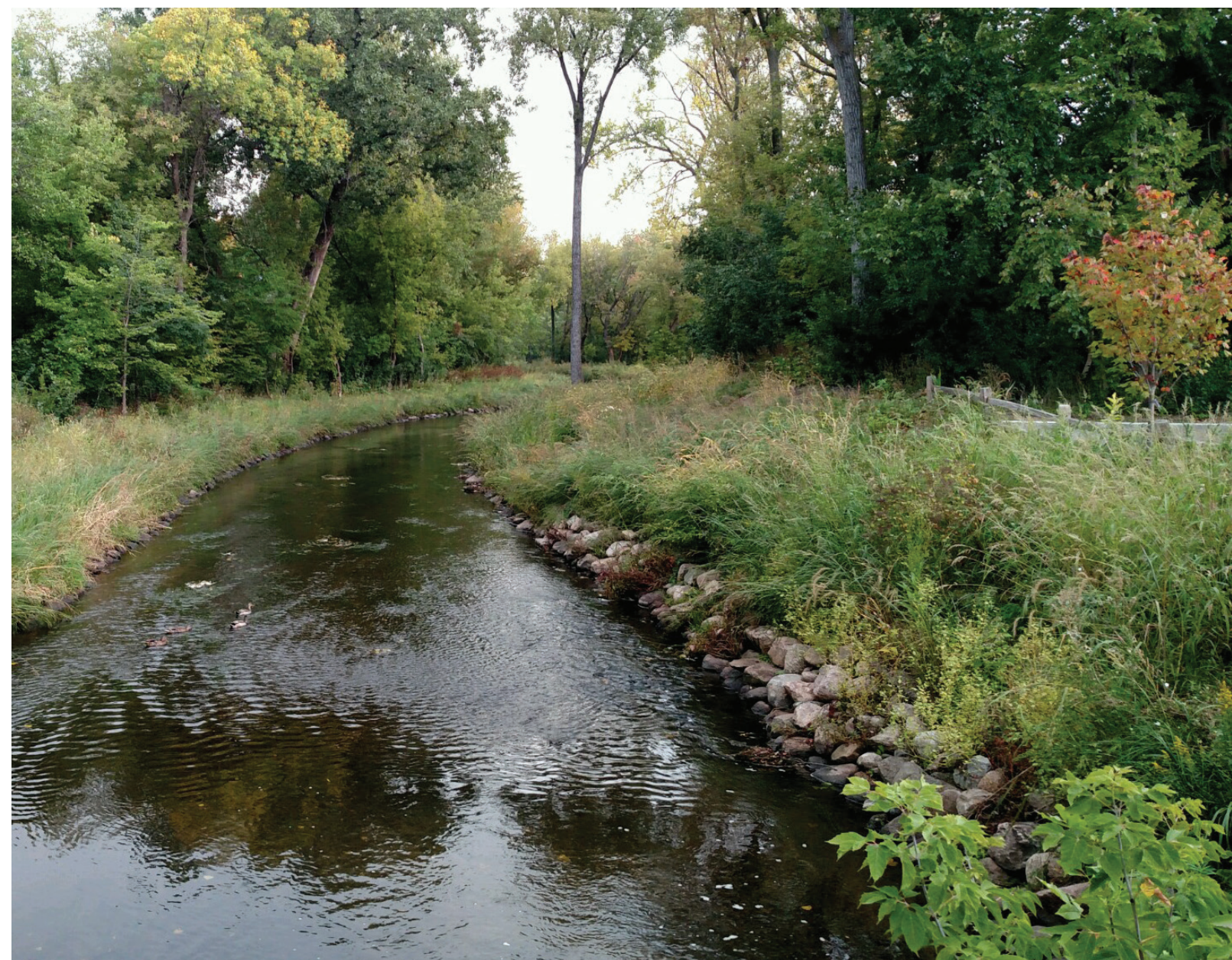
Riprap Toe with Grading to Improve Floodplain Connection - Two years after construction
