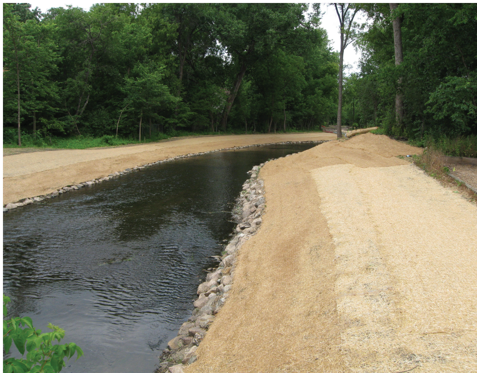
Riprap Toe with Grading to Improve Floodplain Connection - Post construction
