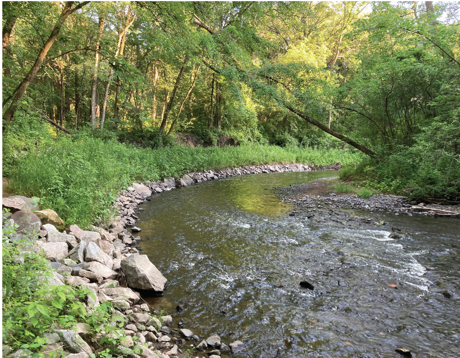
Vegetated Reinforced Soil Stabilization (VRSS) with Riprap Toe
