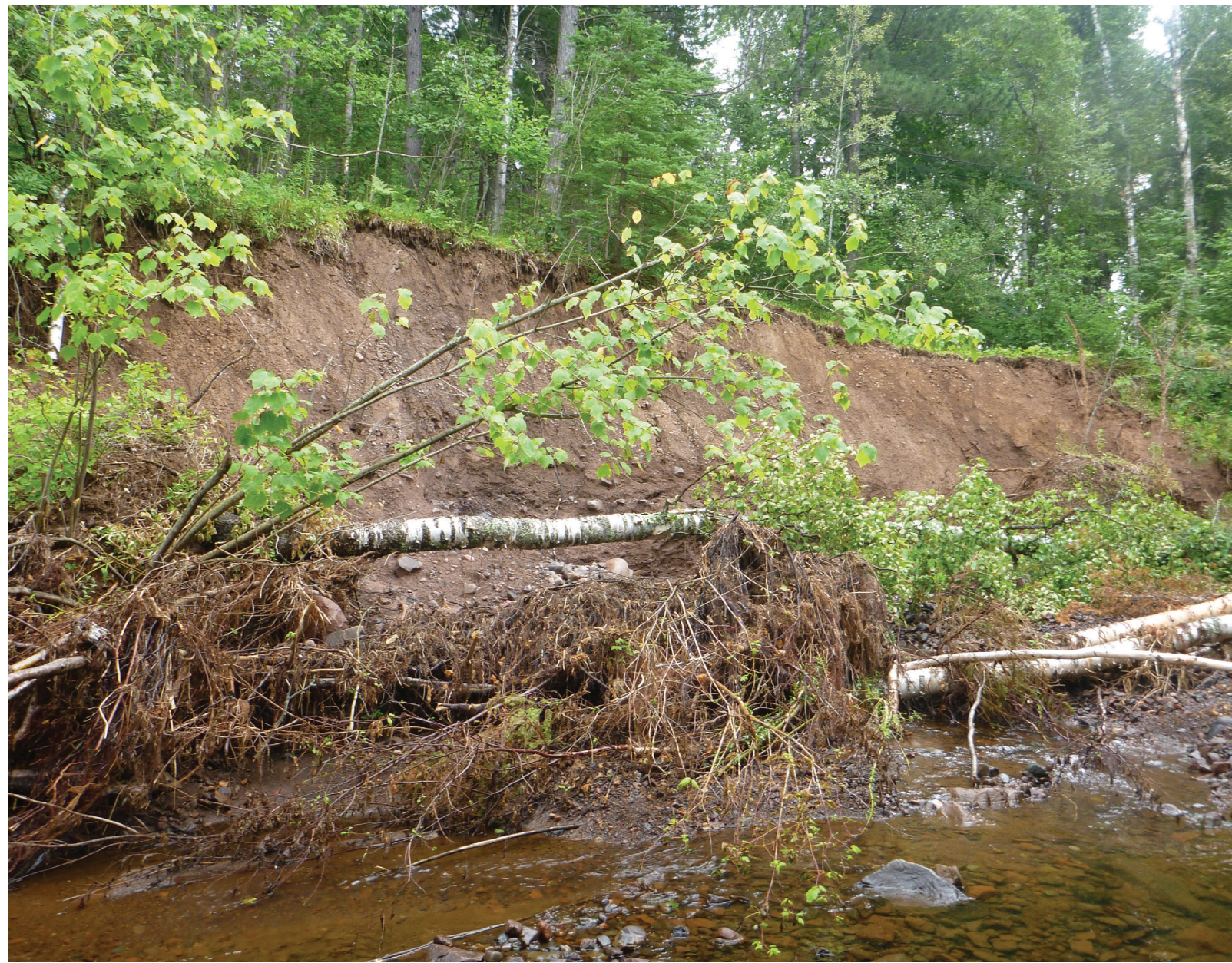
Before - steep, eroding bank with unstable toe
