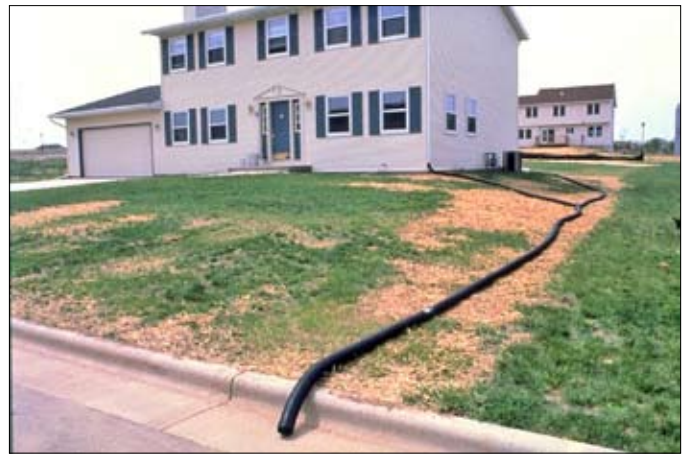
Extenders can direct water from your roof gutters to paved or grassed areas. Be aware that direct discharge, like this, to storm sewers may not be allowed in your area. Be sure to check with your local authorities.
