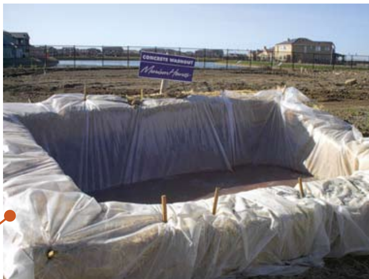
Photo 1: Well-maintained and labeled concrete truck washout
